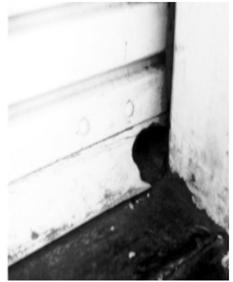
Fig. 4c. Large hole gnawed by Norway rats in weather strip on the base of a warehouse door.
