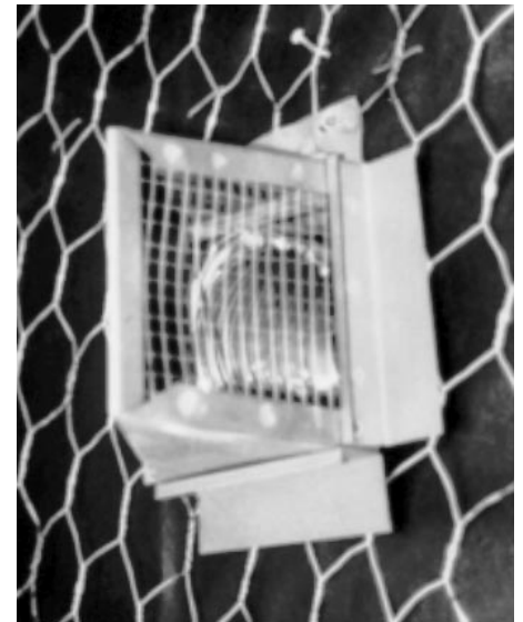
Fig. 26. A side wall exhaust vent with 1/4-inch hardware cloth.
