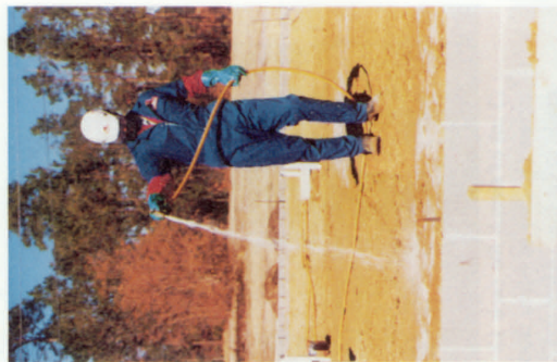
Figure 20. — Chemical treatment of the fill material prior to pouring a concrete slab protects wood in the building from termite attack.
