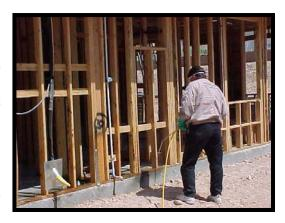
Borate based pesticides used in Nevada for the pre-treatment of wood upon slab type foundations is applied directly to wooden members, utility penetrations and in some cases concrete surfaces as specified by the pesticide label. The use dilution of these pesticides is applied as a liquid solution to all exposed wood surfaces "to a point of wetness" by sprayer, brush, or roller.
