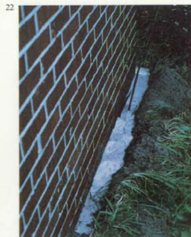
Figure 22. — Application of a chemical to soil around the foundation.
