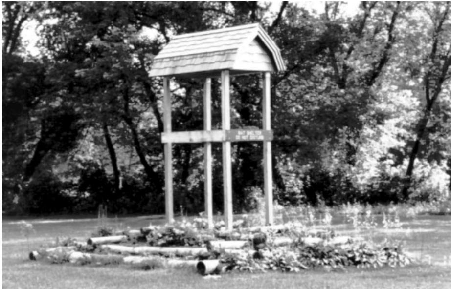
Fig. 16. One of five bat houses constructed to provide an alternative roost for bats excluded from nearby structures.
