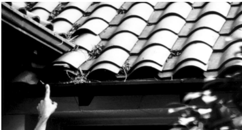
Fig. 15. Open ends of tile roofs may allow bat entry and provide roosting sites.
